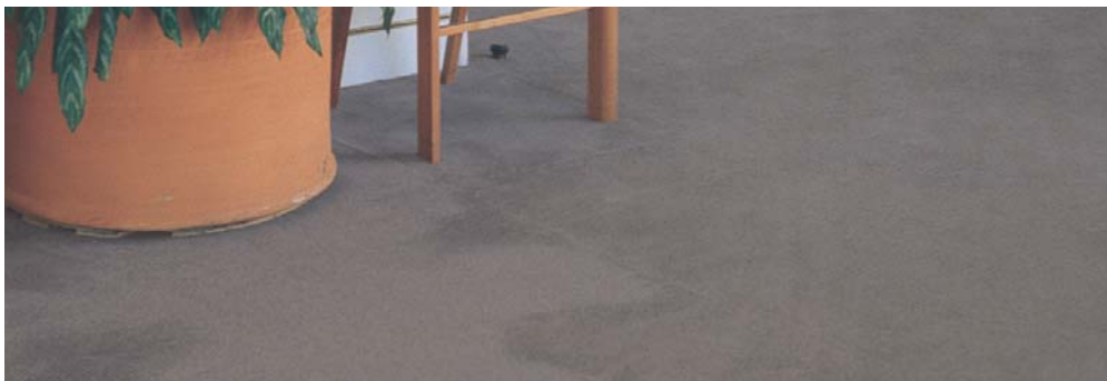
Photograph C - Watermarking, pooling and puddling
